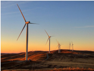
(c) Wind turbines
